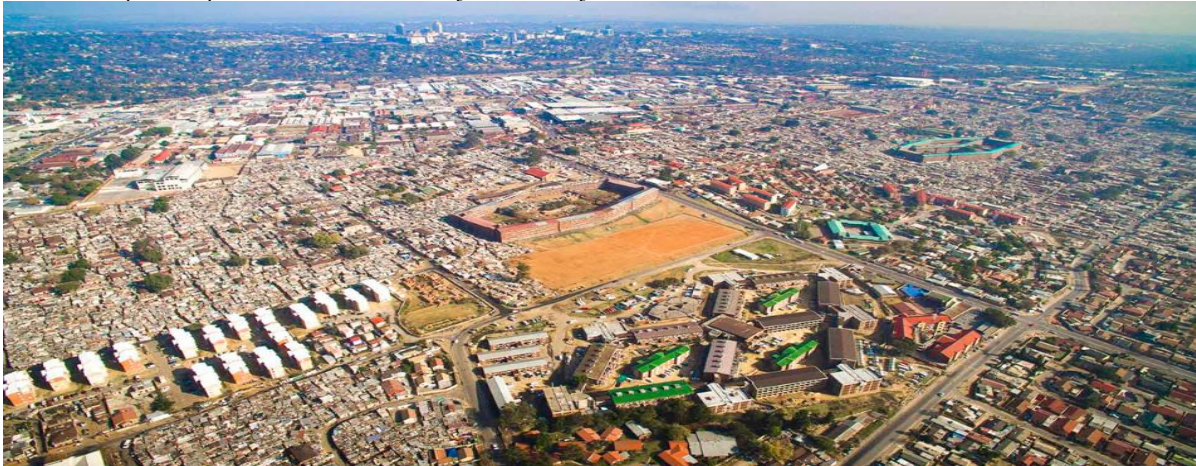
Figure 5: Aerial view of Sandton and Alexandra (Johannesburg)
